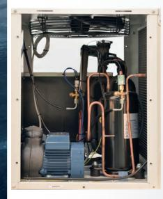
The steel frame and panels are externally powder coated, making QBE suitable for outdoor and weatherproof installations. All fasteners are in stainless steel or electro-galvanized. The panels are easily removable allowing access, allowing access inside the unit for maintenance and repair.
